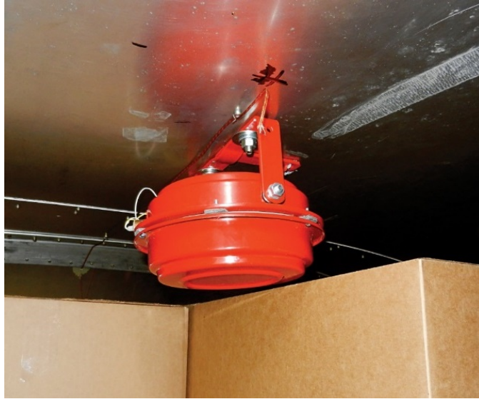
Figure 6.2 – In-container fire suppression system
